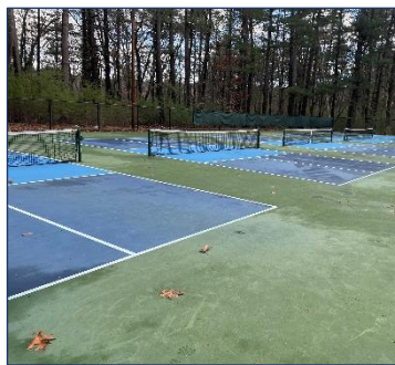
Pickleball courts installed at Recreation Park
