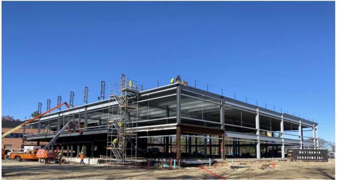
Progress photos of 1 Corporate Drive
