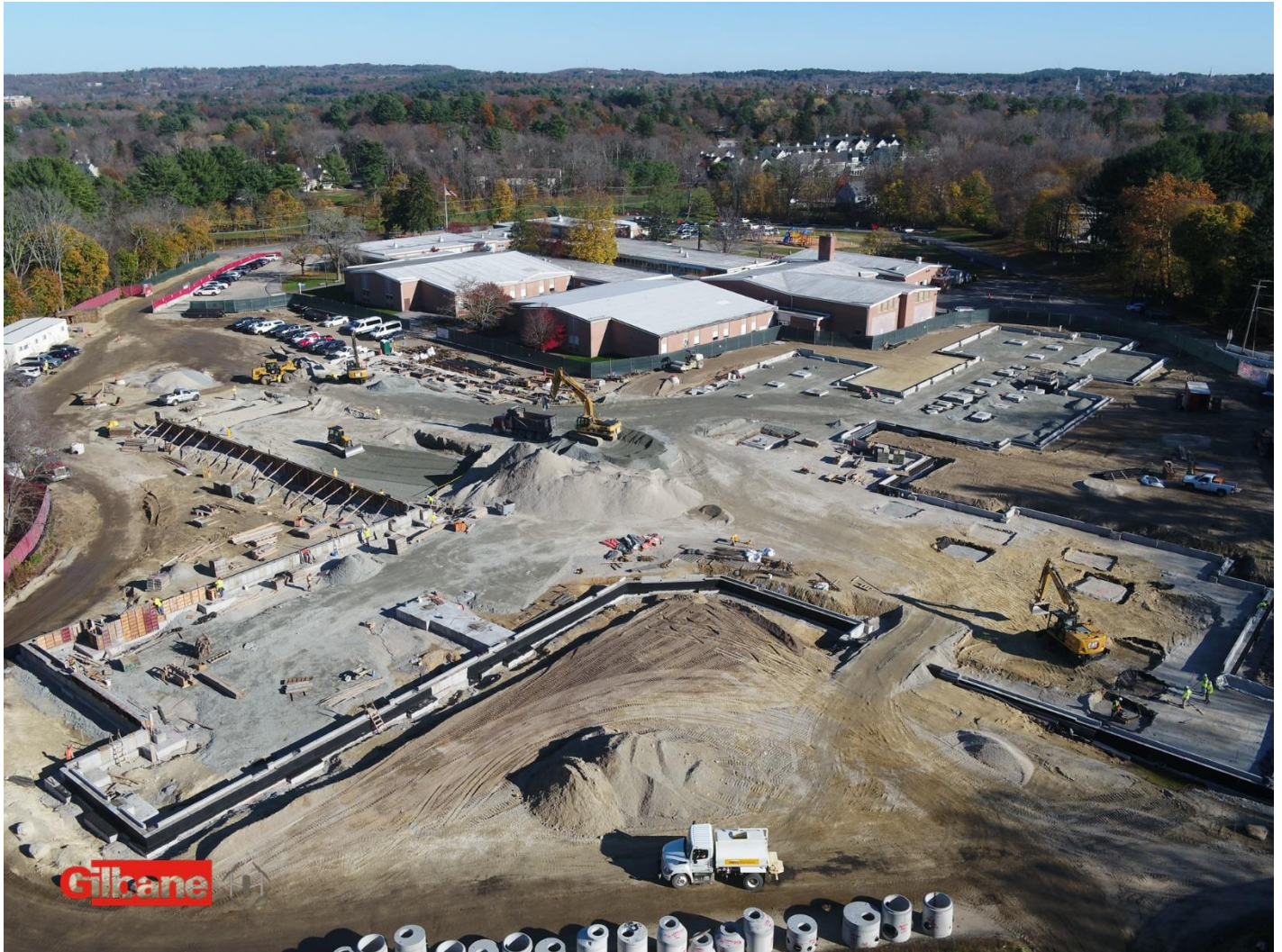
Aerial View of West Elementary School Construction- October 2022
