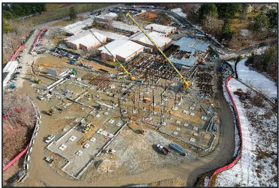
West Elementary and Shawsheen Preschool: Steel framing is being erected in the foreground. West Elementary school is visible at the rear of this photo.
