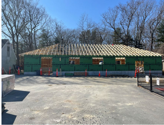
Greater Lawrence Technical School Aviation Building
