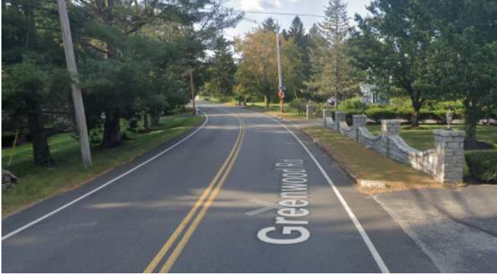
Greenwood Road near Candlewood Drive, looking north
