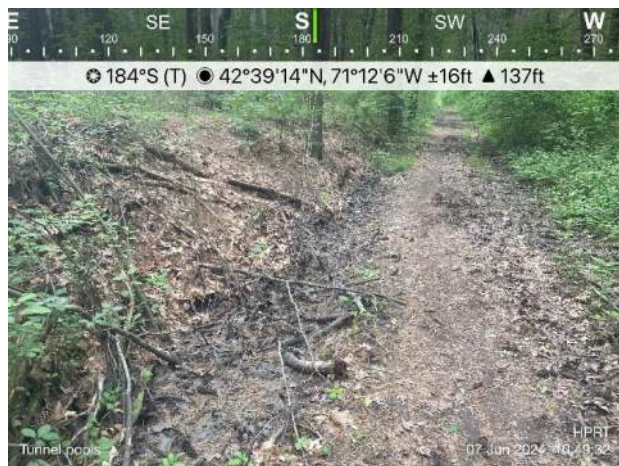
Figure 3: “Tunnel Pool” in ditch.
