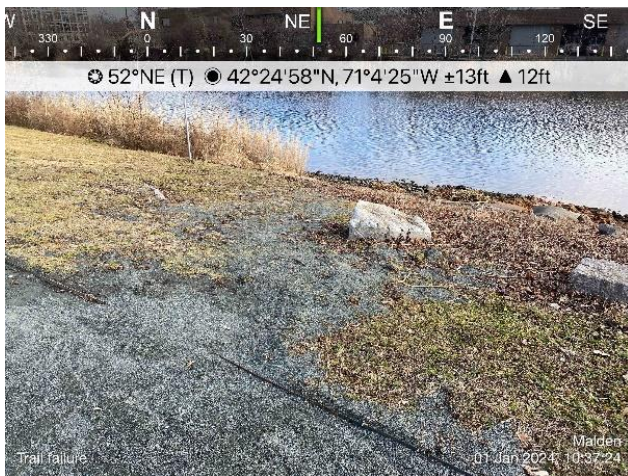
Typical failure profile of stone dust trail surfaces.
