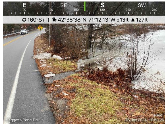
Figure 7. Direct discharge of untreated Haggetts Pond Road stormwater.
