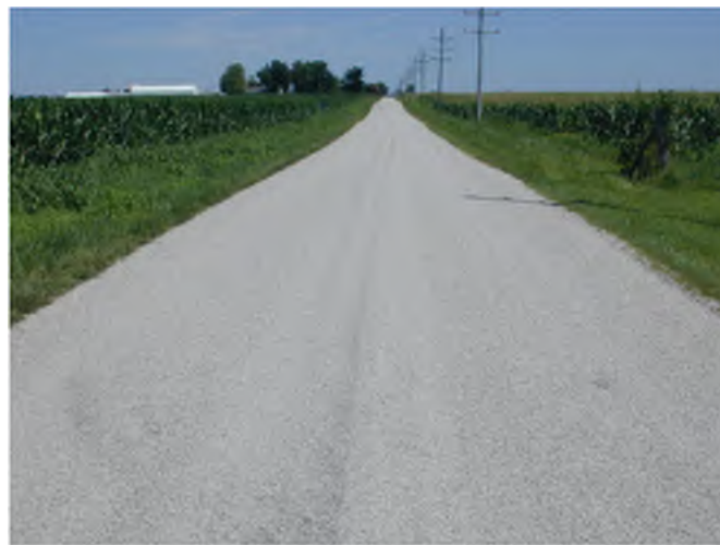
Fig. 4. Newly finished chip seal impervious roadway.
