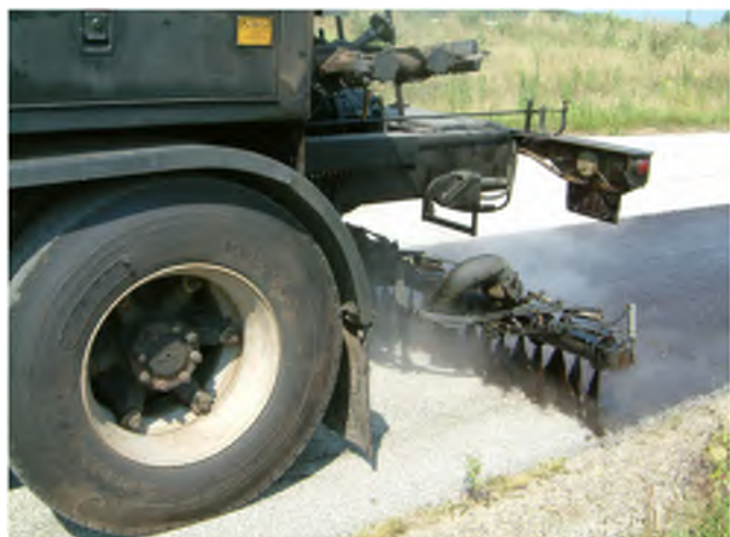
Fig. 2. Asphalt emulsion sprayed on the prepared road during chip seal process.
