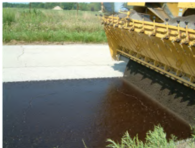
Fig. 3. Aggregate stone chips are spread on the freshly sprayed road.
