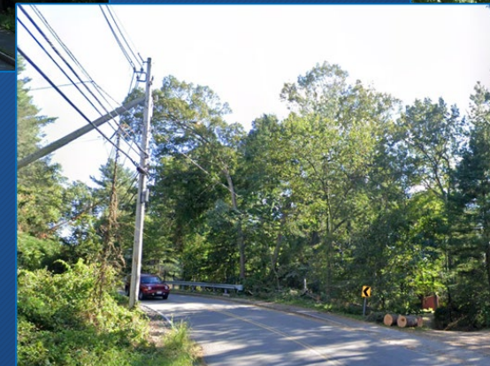
Abrupt Horizontal and Vertical Curvature
