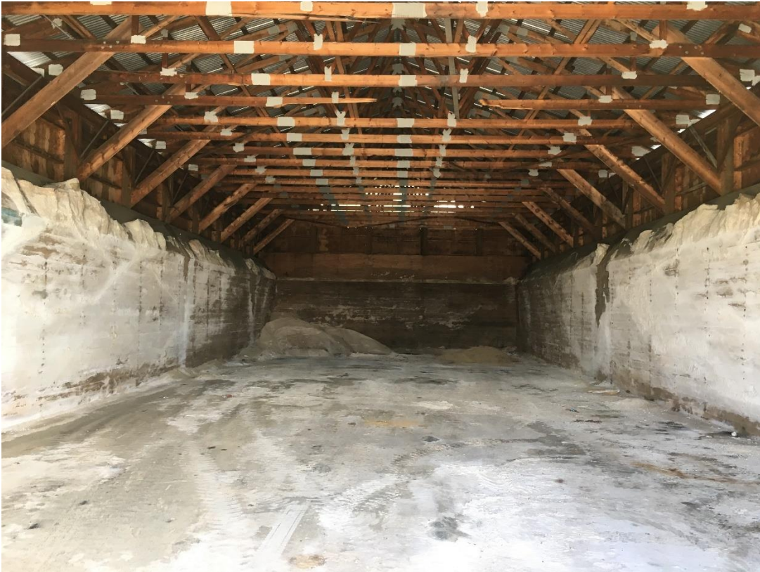
A view of the interior portion of the salt barn building
