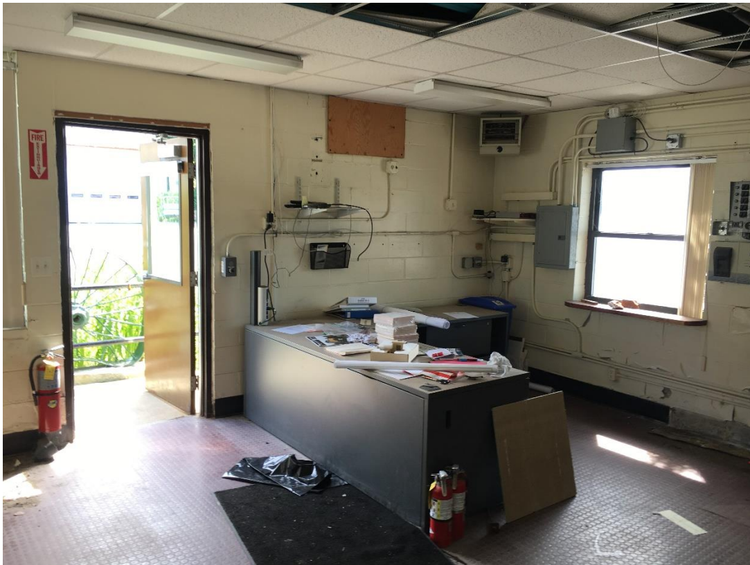
A view of the office area within the Highway Department building
