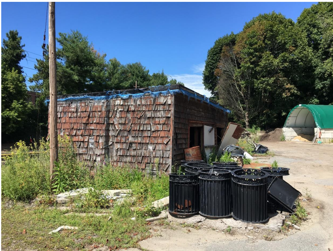
A view of the shed building as viewed from the south
