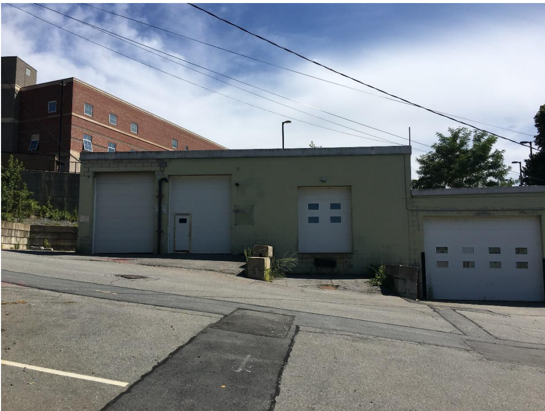
A view of the eastern portion of the Water/Forestry Department building, facing south
