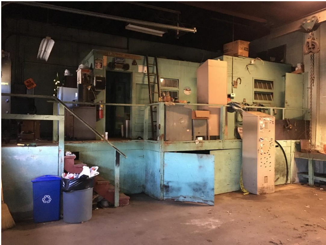
A view of the office/kitchen area within the Water/Forestry Department building
