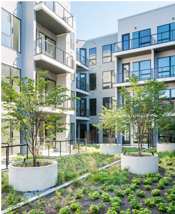
Port 45 – Green Roof
