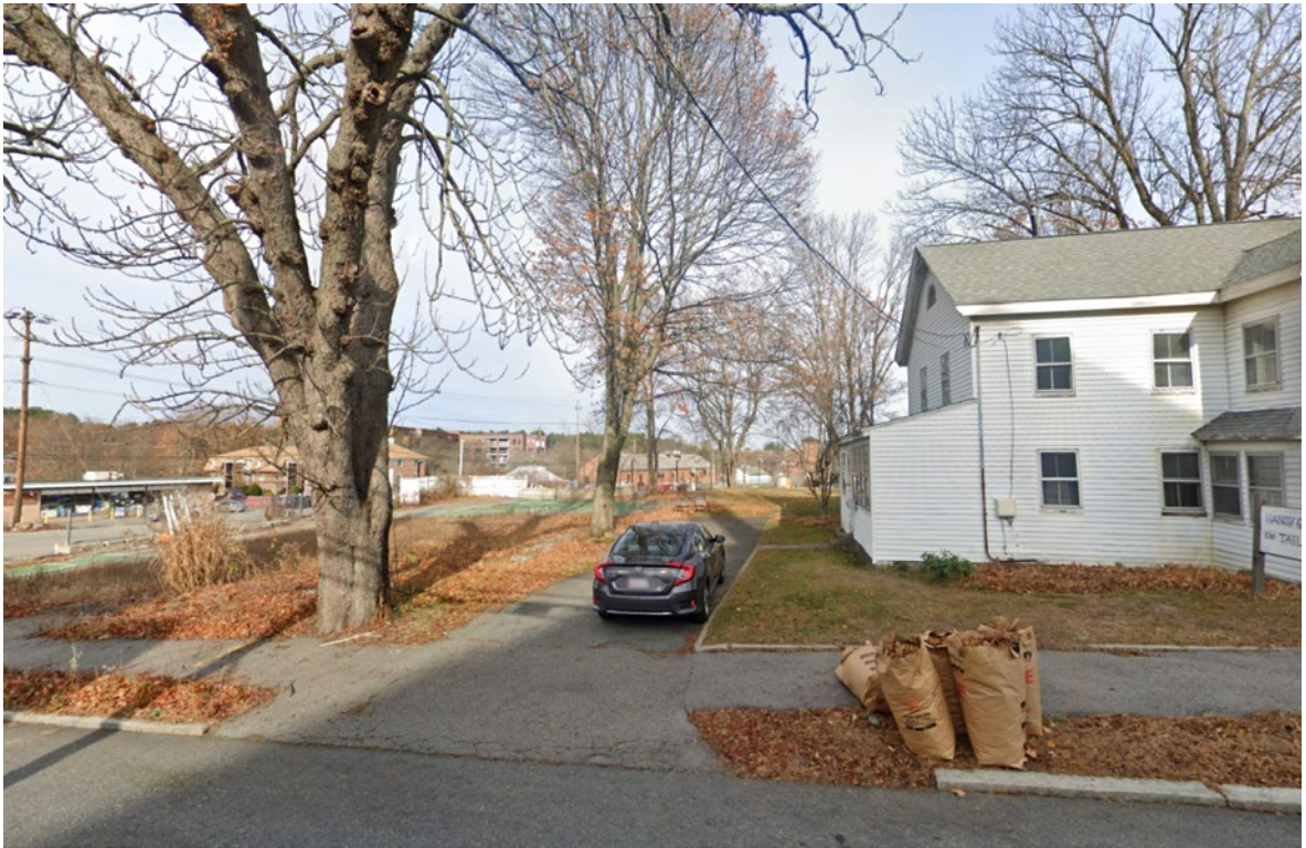
1- SITE FROM PEARSON ST - SOUTH VIEW
