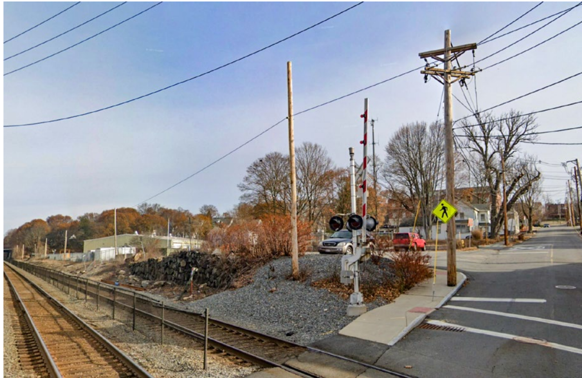
1- SITE FROM PEARSON ST - SOUTH WEST VIEW
